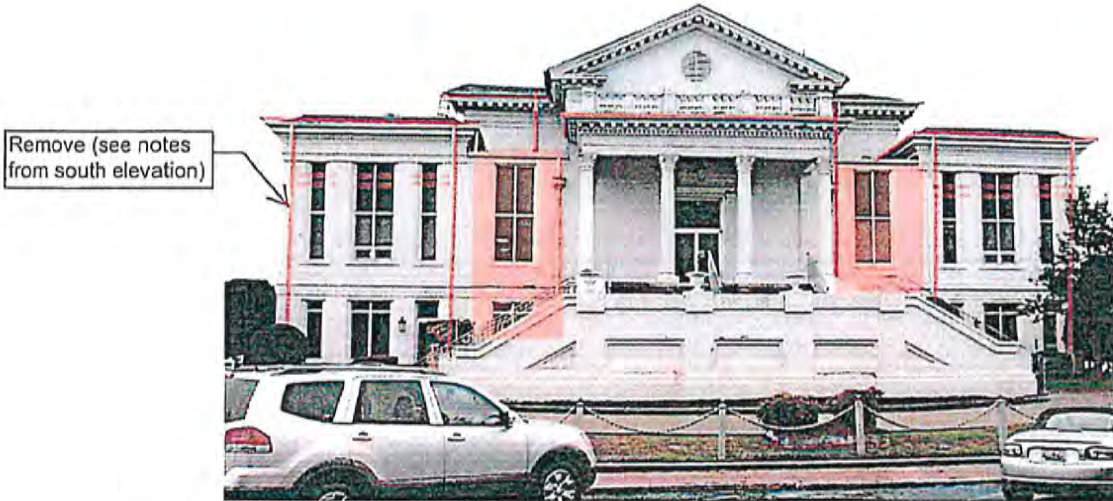
Figure 8 – North Elevation (from the NE) Today
