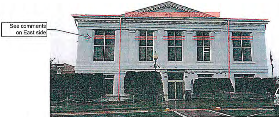
Figure 10 – West Elevation Today
